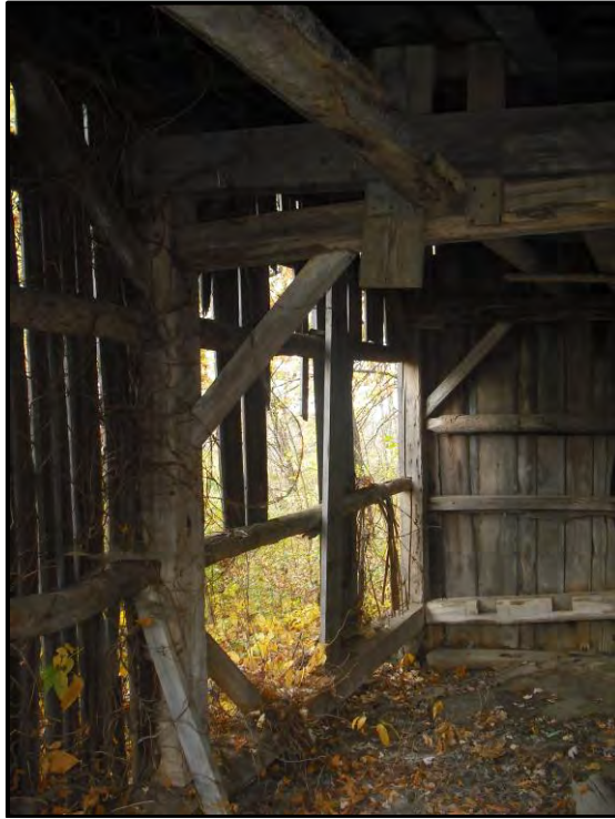
FIGURE 8. FEATURE 2 AT SITE 33LN0284; FACING SOUTHEAST
