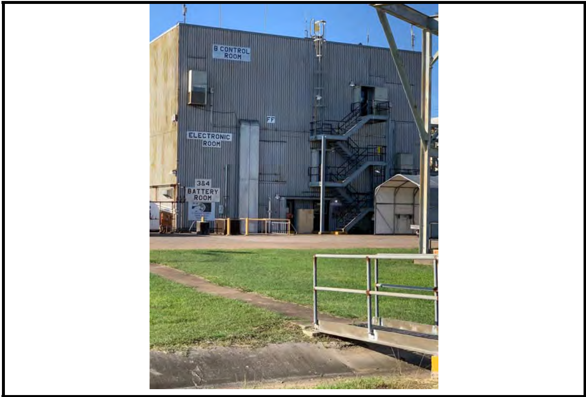
Photo 3: B Control Room and Instrumentation & Control Shop, facing south.
