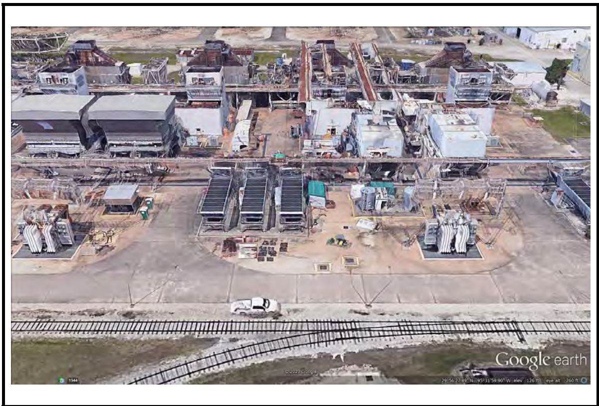
Photo 5: Gas Turbines 31, 32, 33, and 34, facing north.
