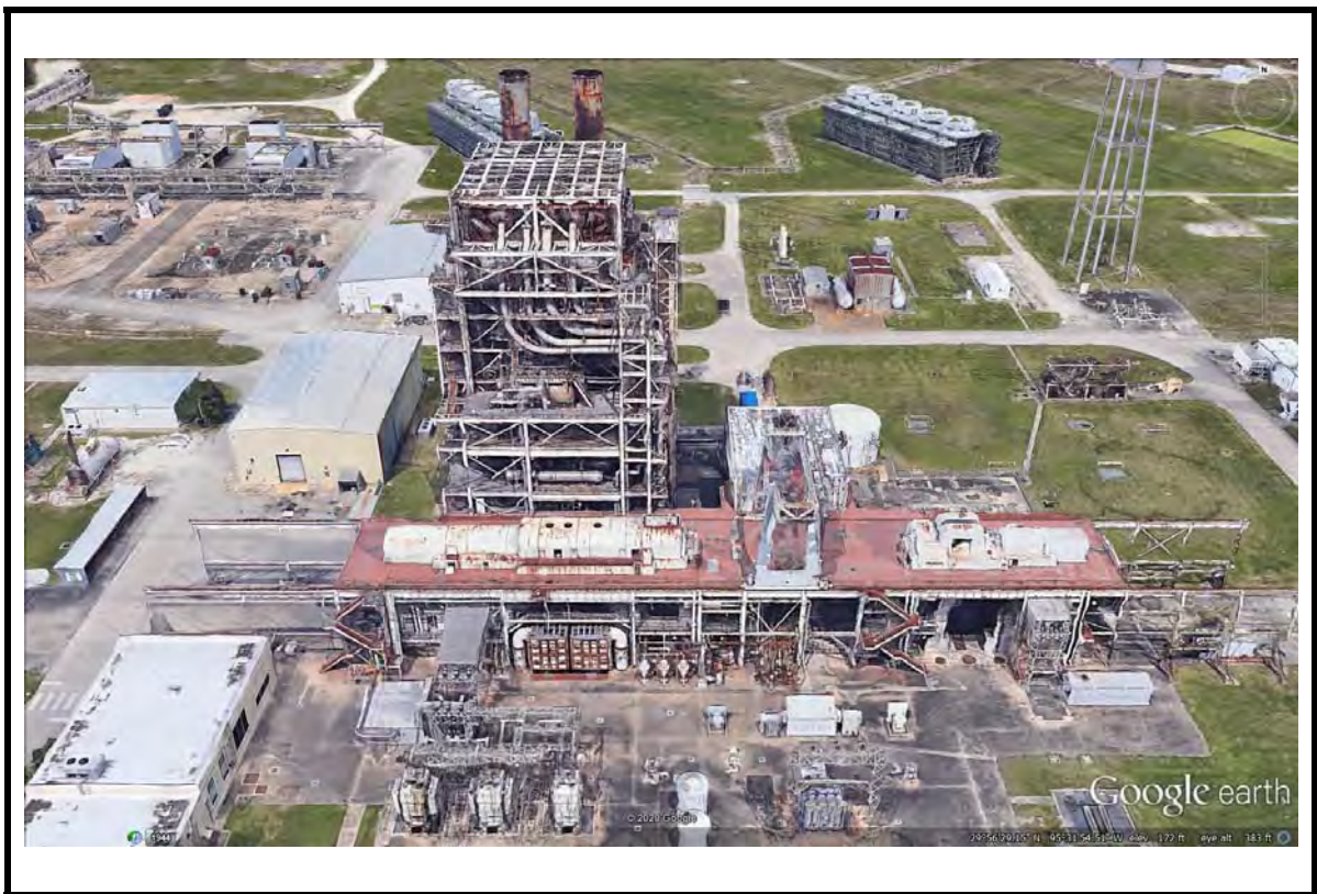
Photo 9: Generating Units 1 & 2 and associated Cooling Towers (all retired), facing north.
