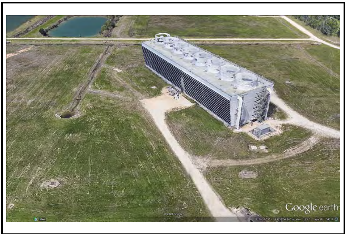
Photo 11: Cooling Tower for Units 3 & 4, facing northeast.
