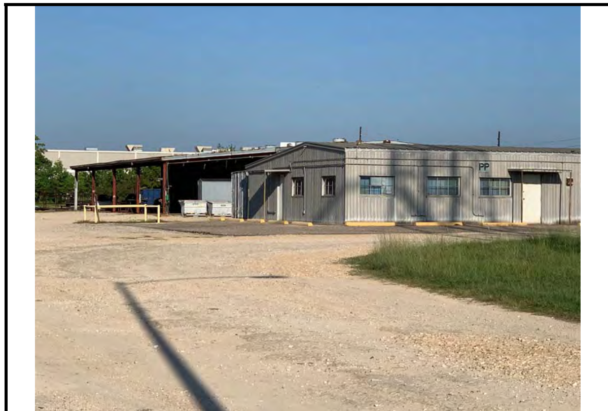
Photo 10: Contractor Building and Weld Shop, facing northwest.
