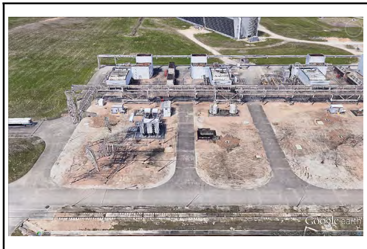
Photo 8: Gas Turbines 54, 55, and 56, facing north.
