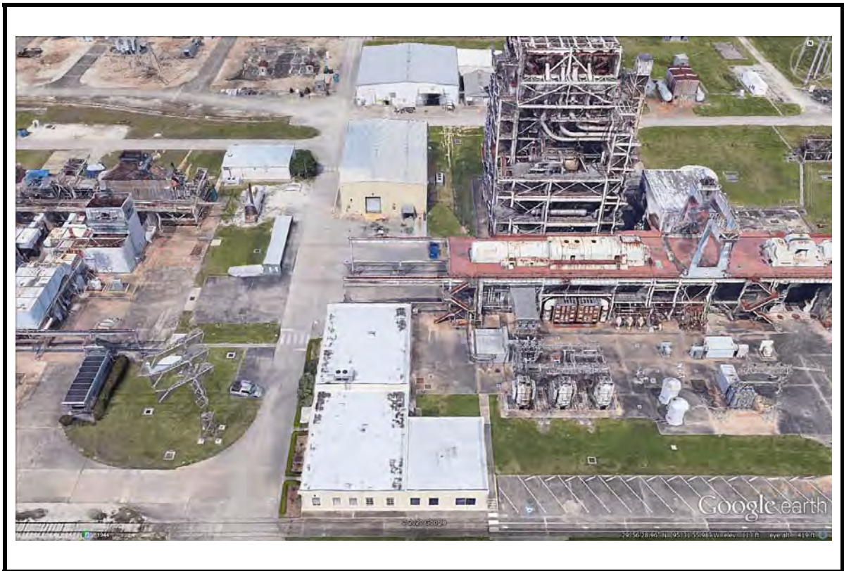
Photo 13: Warehouse, Mechanic Shop, and Administrative Building, facing north.
