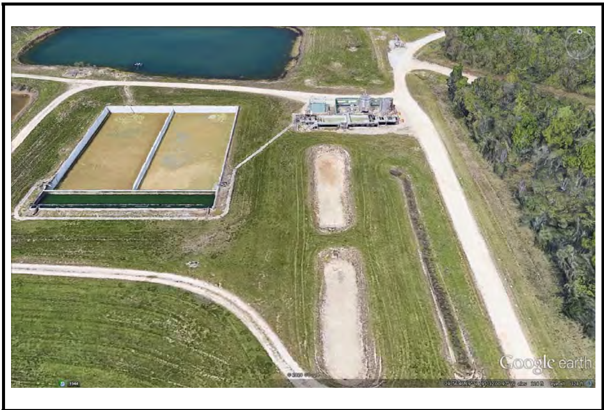
Photo 4: Chemical Waste Treatment System, facing north.
