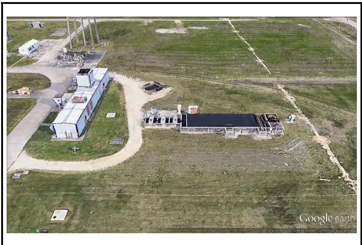
Photo 12: Gas Turbine 1 and Floor Drain Treatment System, facing north.
