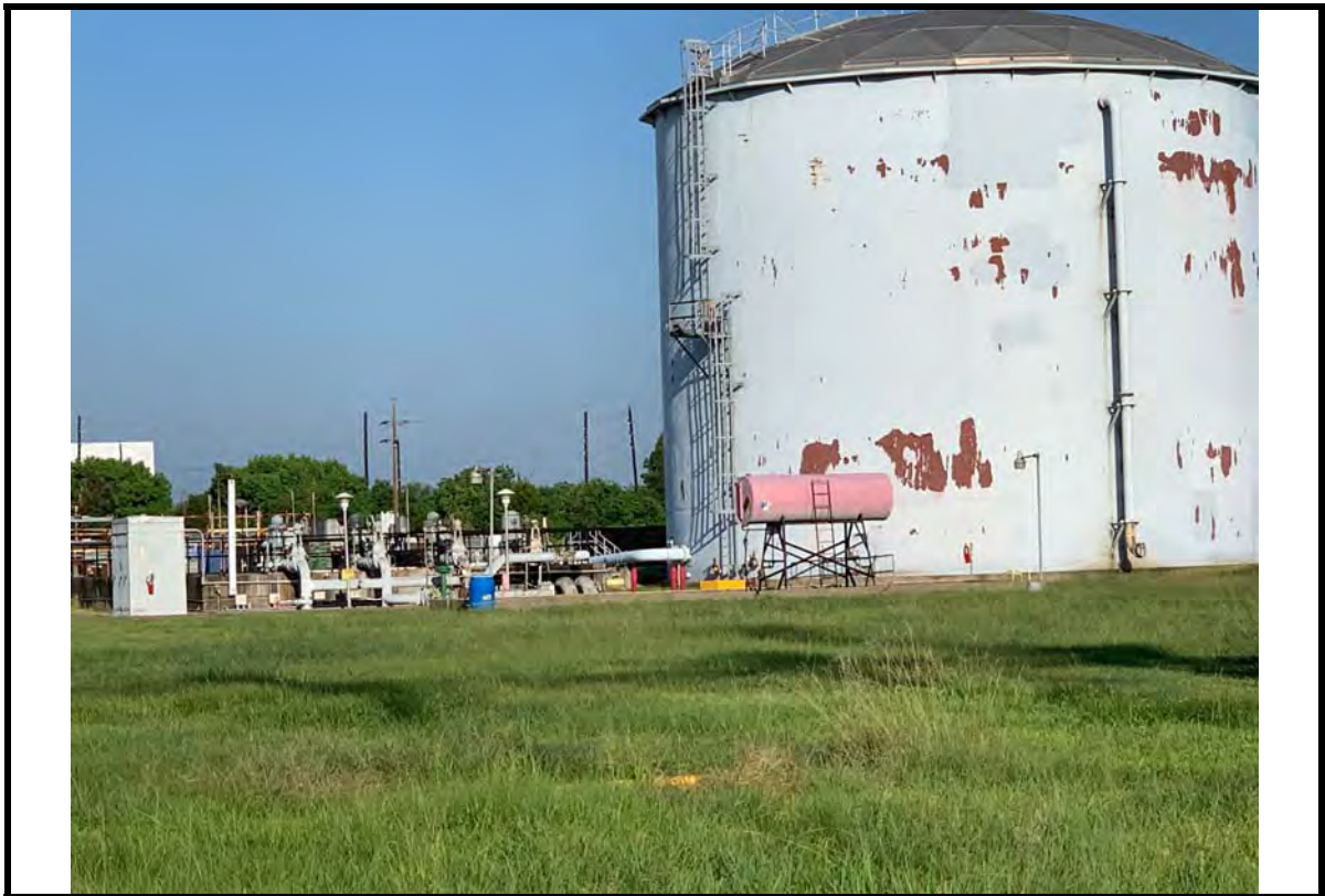
Photo 2: Settling Basin and Water Storage Tank, facing west.
